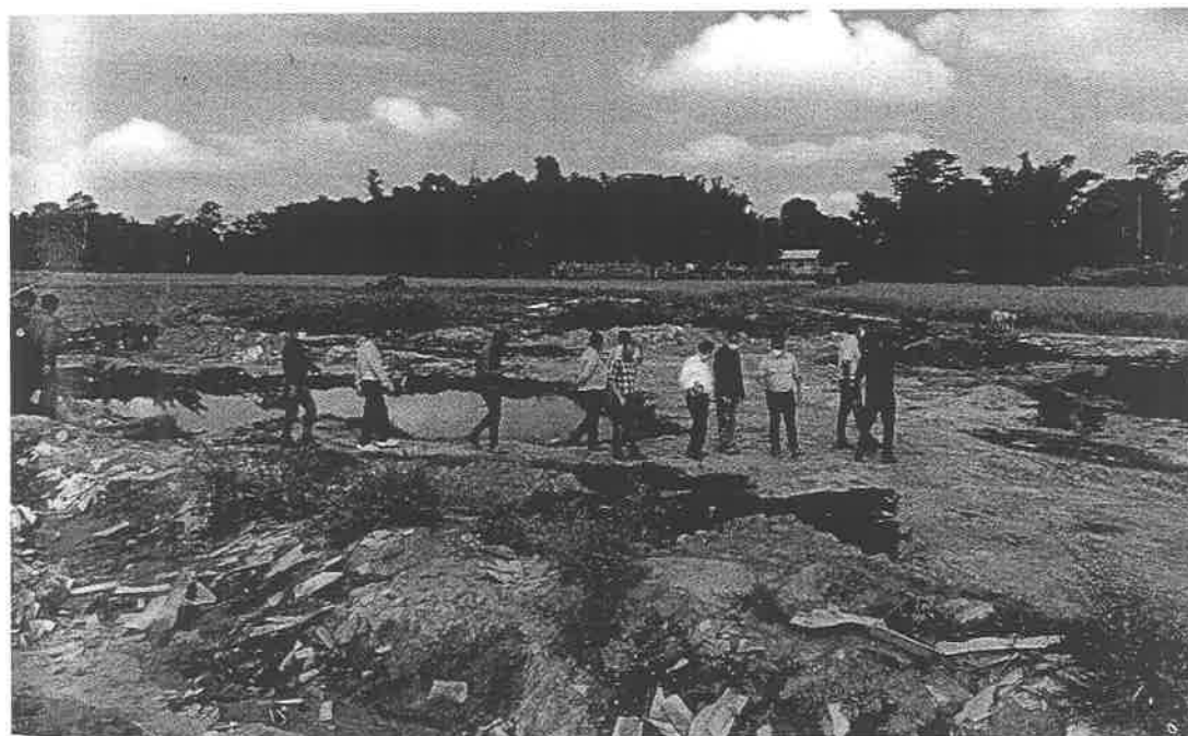
Figure 4: Committee at BGN#5 accident site on Oct 8, 2021
